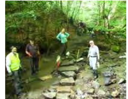
concrete in the stones, in the dry portion, so hopefully they stay in place despite any future flooding. We are also looking to see if it is feasible to make some steps on the steep slope at the exit from the stepping stones into Jagger Park Woods
